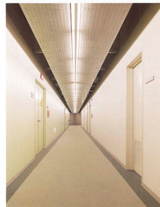
▲3階廊下 Corridor on the 3rd floor.
