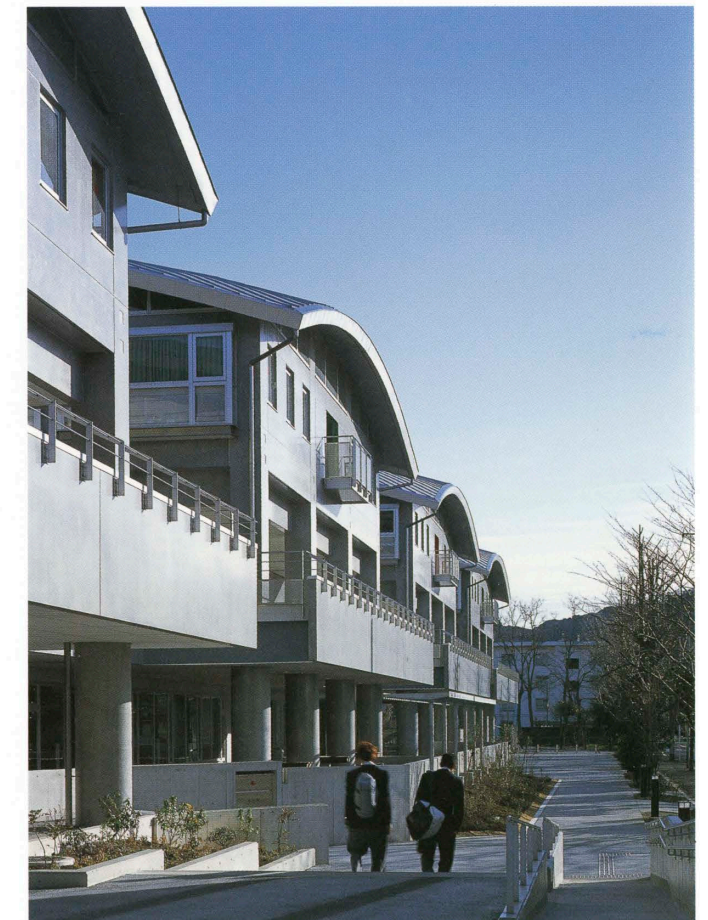
校舎棟西側 West side view of schoolhouse.
