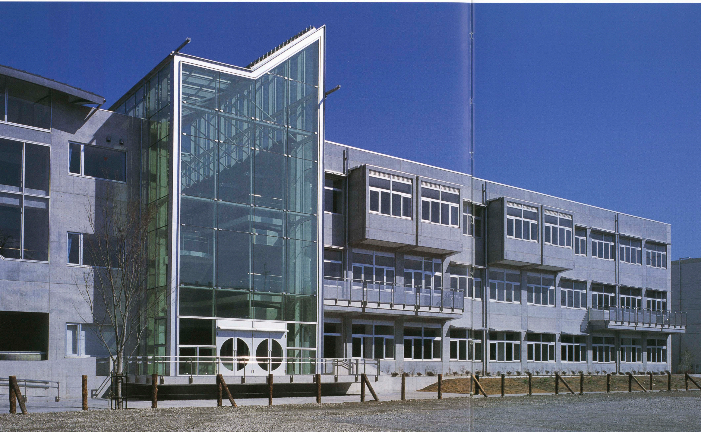
校舎棟南側外観 South exterior view of schoolhouse.
